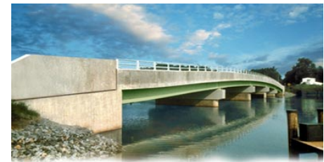
Scotchman's Creek Bridge—Cecil County, Maryland
