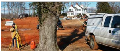
Condo & Easement Plats/Construction Stakeout Suffield Meadows— New Baltimore, Virginia
