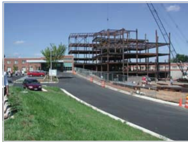
Boundary/Topo/Utility Surveys/Const. Stakeout Fauquier Hospital -- Warrenton, VA
